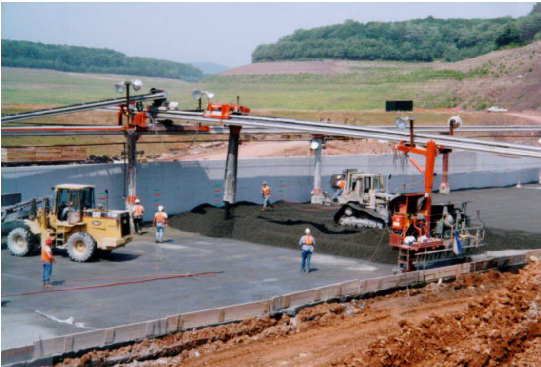
Figure 6-2. Conveyor system with mobile side discharge belt
